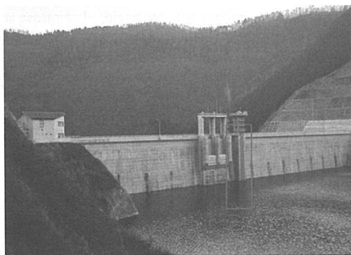
Photo 3. The intake of the Tsuchimurogawa hydropower plant from the upstream of the Kazunogawa dam.
