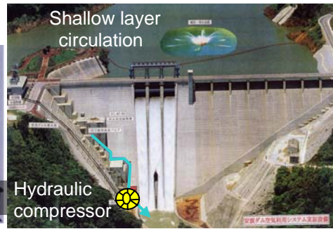
Fig. 4 Dam Air-energy System in Aha dam
