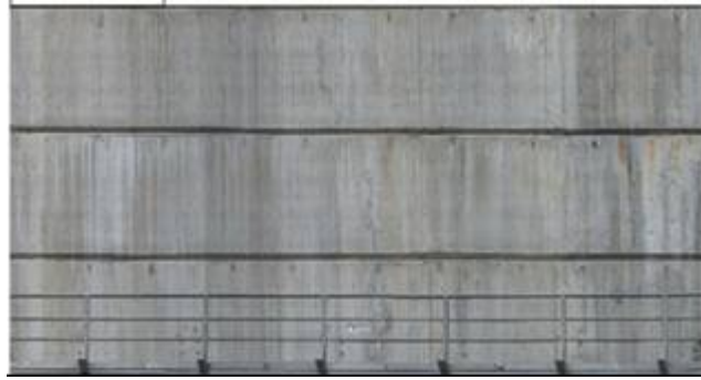
Fig. 8 Example of image joining (joining of 150 images) Exemple du couplage des images
