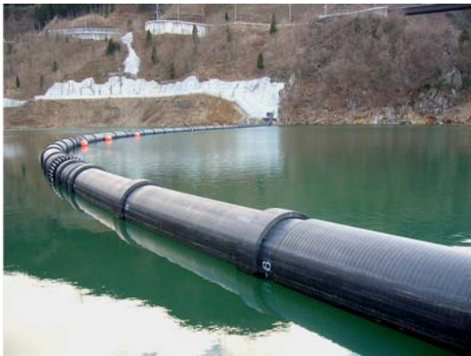
Fig.11 Suspended Pipe Section (1) (Before Submerging)
