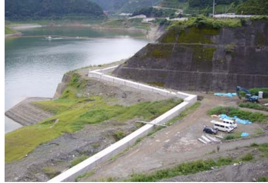
Fig.10 FRPM Pipe Section (2) (Completed with Concrete Cover)
