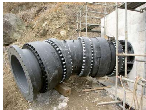
Fig.14 Suspended Pipe Section (4) (Rotation Joint)
