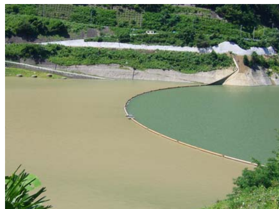
Fig.3 Floating Turbidity Curtain
