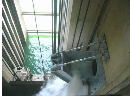
Fig.16 Outlet (2) (Inside the Intake Tower)
