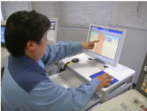
Fig.17 Remote Control System (Operation Room)
