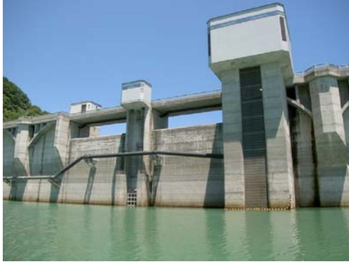
Fig.15 Outlet (1) (Intake Tower)
