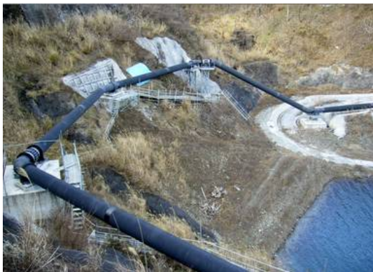
Fig.7 Steel Pipe Section (1)
