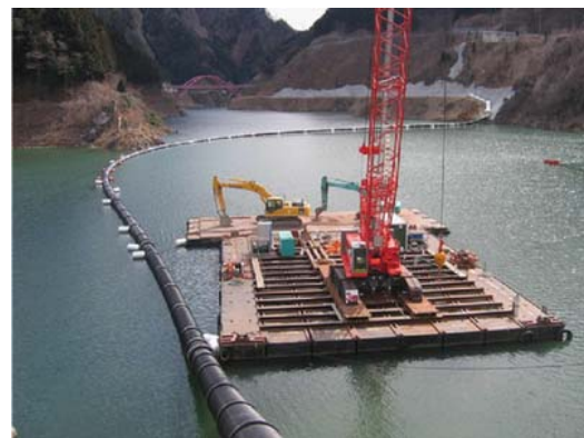
Fig.12 Suspended Pipe Section (2) (Construction Work)
