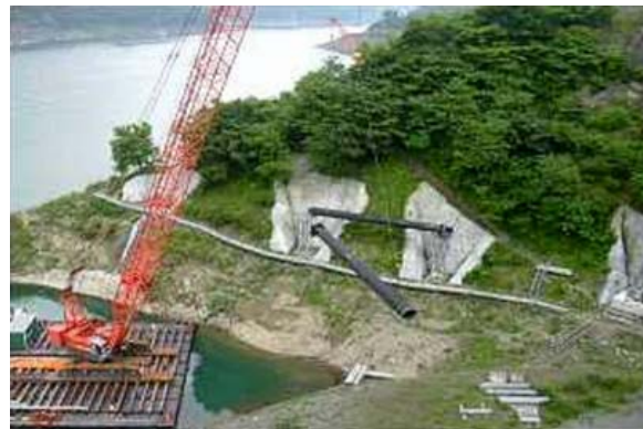
Fig.18 Construction Work (A Crane on the Pontoon)
