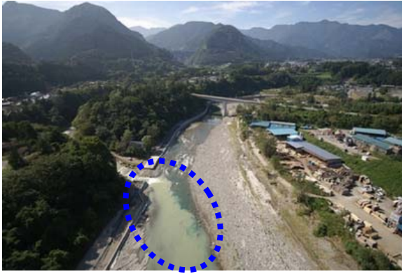
Fig.20 Before Operation (28 Sep. 07) (Turbid Water Flows into the Main River)
