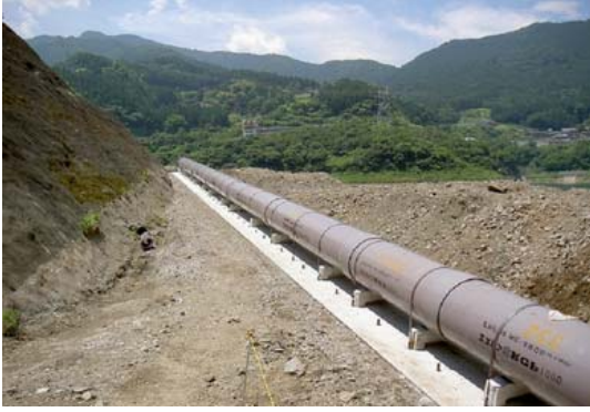
Fig.9 FRPM Pipe Section (1) (Under Construction)
