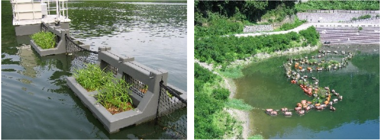
Photo 8. Vegetated Floating Island Type Boom and Floating Island Reusing an Old Boom
