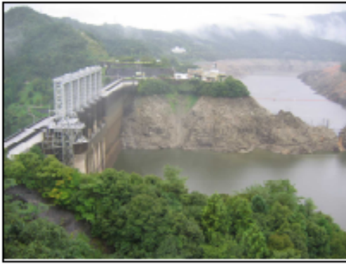
Fig. 17 Sameura Dam Before and After Flood Control at the Time of Typhoon 14 in 2005 (Secured storage rate: 0% (before flood control as shown in left photo), 100% (after flood control as shown in right photo))
