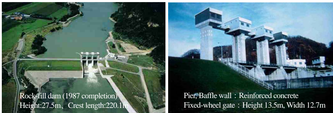
Fig.1 Spillway analyzed in this study
