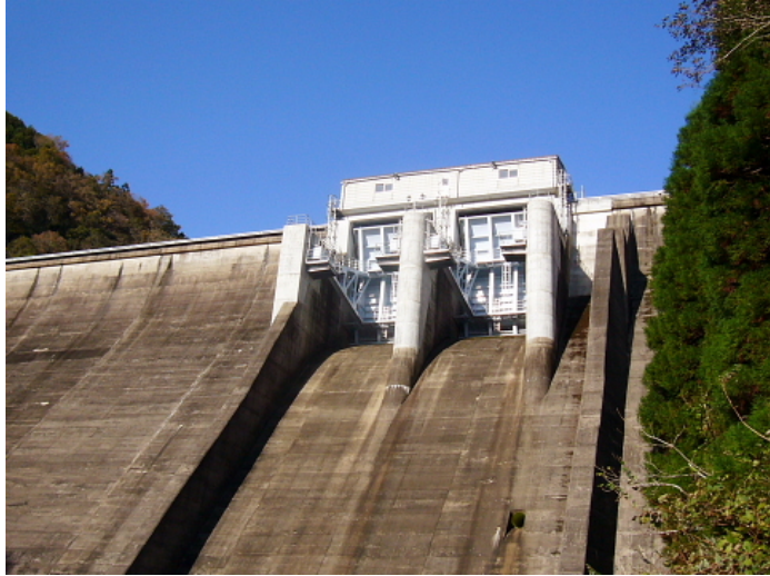
Picture 1 Sabagawa dam (reconditioned gates)
