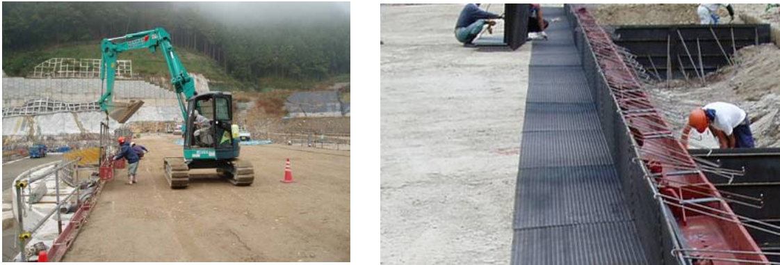
Figure-7 Moving H-shaped Steel Shuttering and Installation of Steel Meshes Shuttering.
