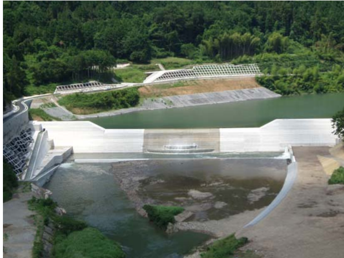
Figure-2 View of Completed Kawai Dam
