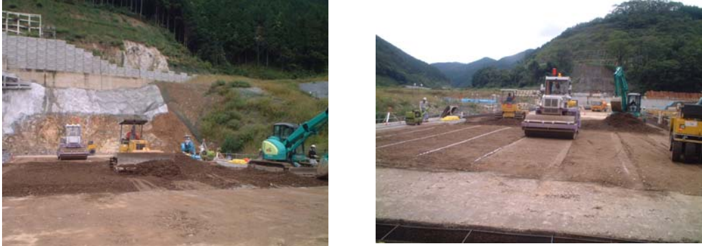
Figure-6 Spreading of CSG and Compaction in General Area
