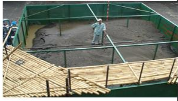
Photo 2 Accumulated sediments in return tank
