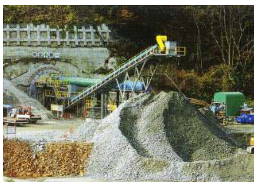
Photo 7 Removal of Excavated Material Gravats issues des fouilles
