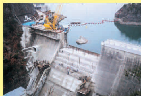
Dismantling the old concrete crown of the main dam structure
