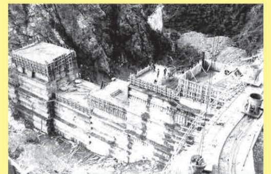
Pouring concrete for the main dam structure
