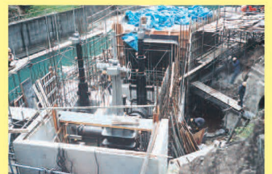
Rebuilding the outflow structure
