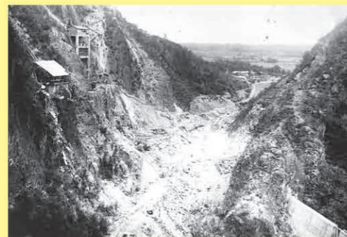
Treating bedrock (looking downstream)
