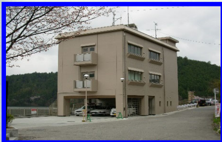
Dam Management Office
