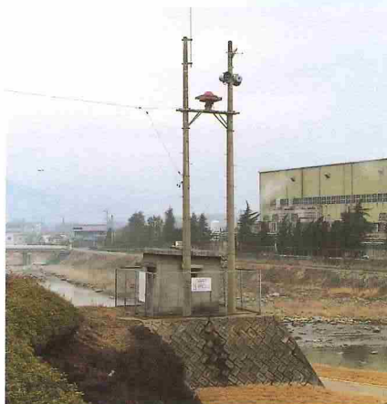
Discharge warning station There are ten stations in the downstream area of the dam to notify discharge from the dam to people who are in or around river.
