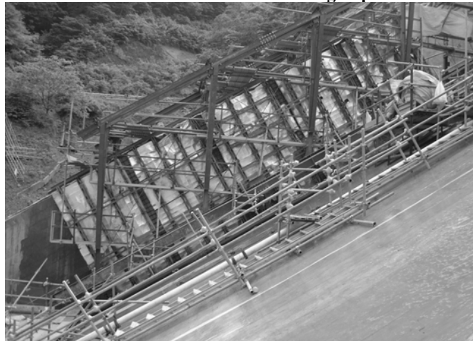
Photo 3. Construction of a Training Wall with Large Sliding Forms
