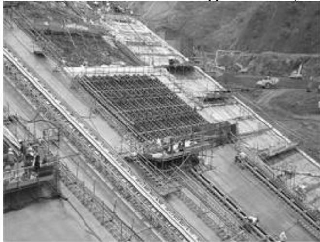
Photo 2. Construction of a Training Slip Forms
