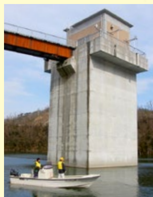
Water withdrawal tower of Tono Dam
