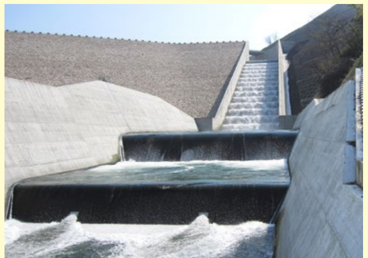
Energy Dissipation by a Cascade Spillway in Tono Dam
