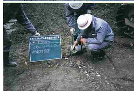
▲Execution of tests on RCD method (upstream cofferdam)
