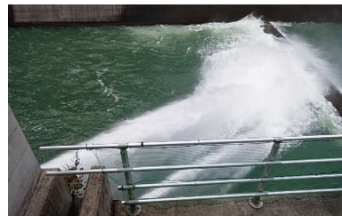
Large discharge conduit 1 jet flow gate [Discharge capacity] 30 m 3 /s
