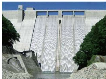
Free overflow type crest [Discharge capacity] 1,800 m 3 /s
