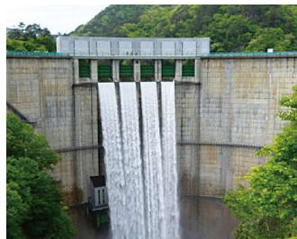
6 roller gates [Discharge capacity] 1,250 m 3 /s
