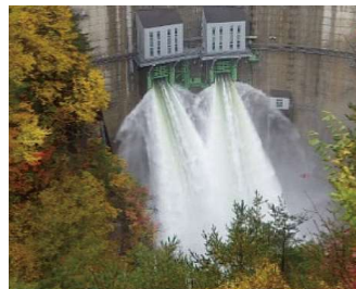
2 high-pressure roller gates [Discharge capacity] 550 m 3 /s
