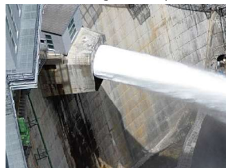
1 Howell-Bunger valve [Discharge capacity] 57 m 3 /s
