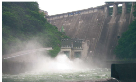
2 high-pressure roller gates [Discharge capacity] 500 m 3 /s
