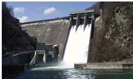
3 two-stage roller gates [Discharge capacity] 3,000 m 3 /s
