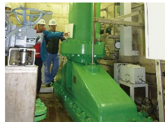
④ The first high-pressure slide gate made in Japan
