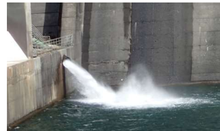
1 jet flow gate [Discharge capacity] 14 m 3 /s
