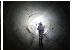
Headrace pipe Headrace pipe carrying 20\text{m}^3 per second (diameter 2.5 m)
