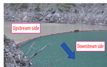
Turbid water diffusion prevention fence at the Kawaji Dam
