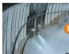
B Two conduit gates Maximum per second discharge rate: 400m 3
