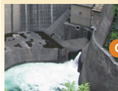
C Two low water outlet facilities Primary maximum discharge capacity per second: 30m 3 Secondary maximum discharge capacity per second: 5m 3
