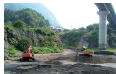
Excavation of sediment deposited at the Kawaji Dam
