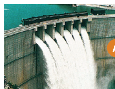
A Six crest gates Maximum per second discharge rate: 4,400m 3
