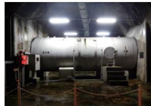
Headrace pipe Headrace pipe carrying 20\text{m}^3 per second (diameter 2.5 m)
