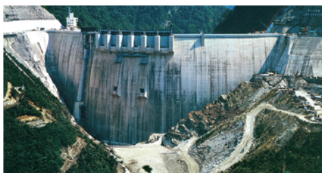
Dam body with a three-dimensional shape similar to a bowl (Upstream side at time of construction)
