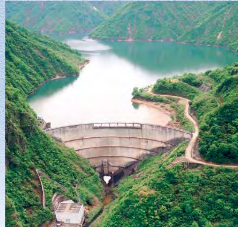
Kuromatagawa No.2 Dam and Power Station
