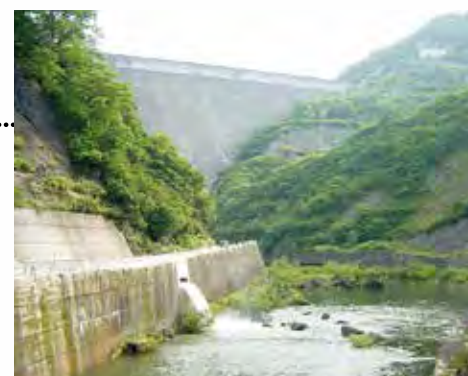
Water discharge from temporary drainage channel (discharged about 200m upstream when power is generated)
