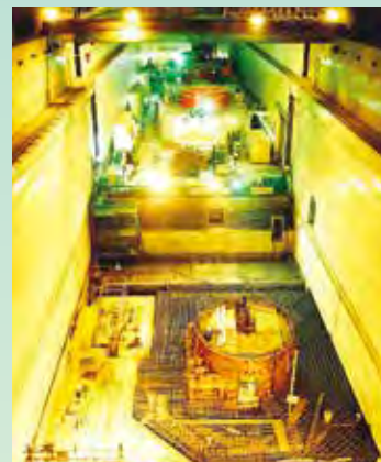
Power Station Work
