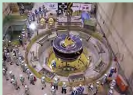
Runner installation Work
