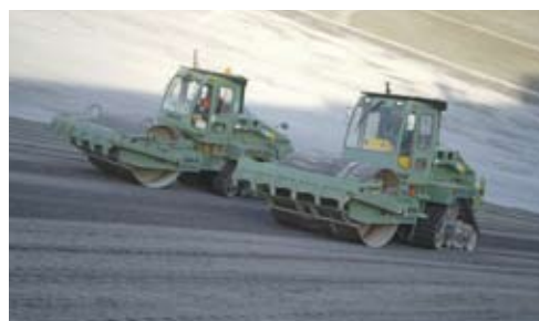
Compaction of base layer
