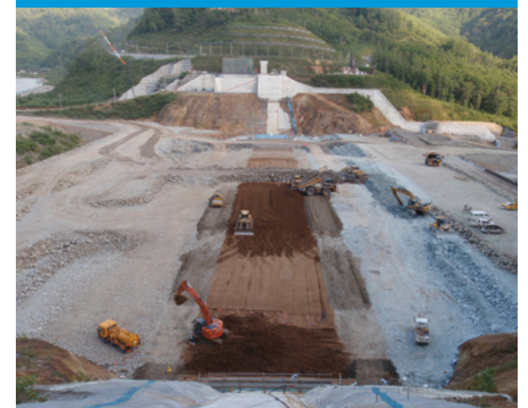
Embankment works of dam body
