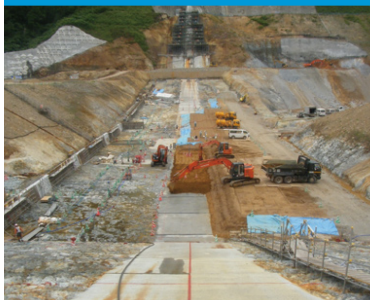
Embankment works at riverbed area
