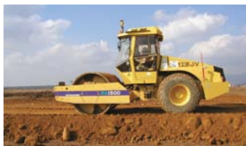
Compaction of dam body embankment
