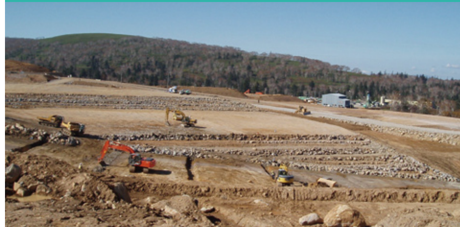
Embankment works of dam body
