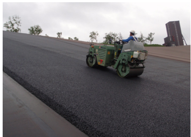
Compaction by a vibration roller
