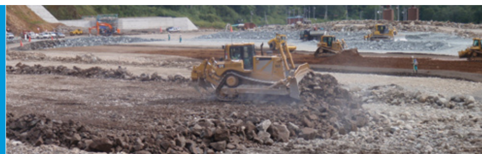
Embankment works of rock material
