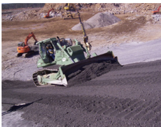
Levelling by a bulldozer
