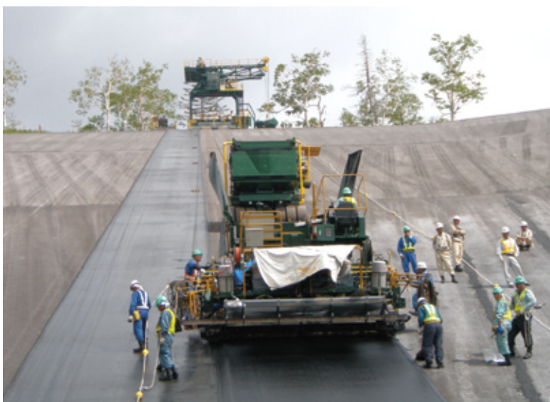
Paving the Lower impervious layer by an asphalt finisher.
