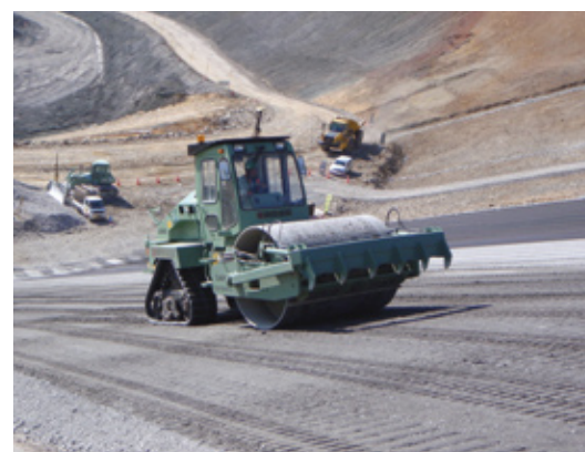
Compaction by a self-climbing vibration roller
