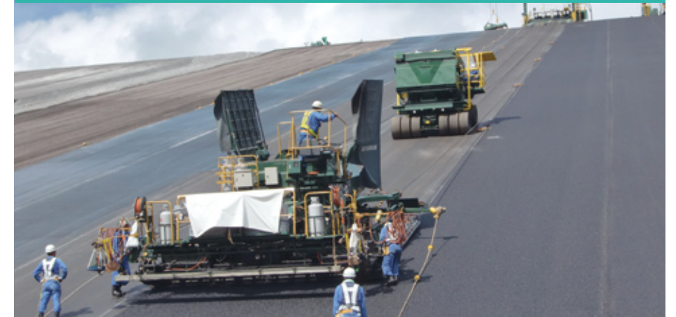
Asphalt facing work
