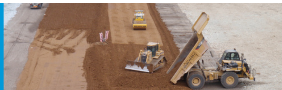
Embankment works of core material
