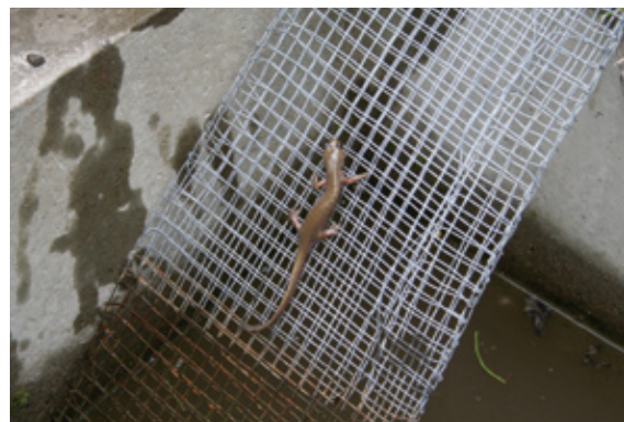
"Haiagaru" (slope: 1 to 0.8, width: 0.2m)
