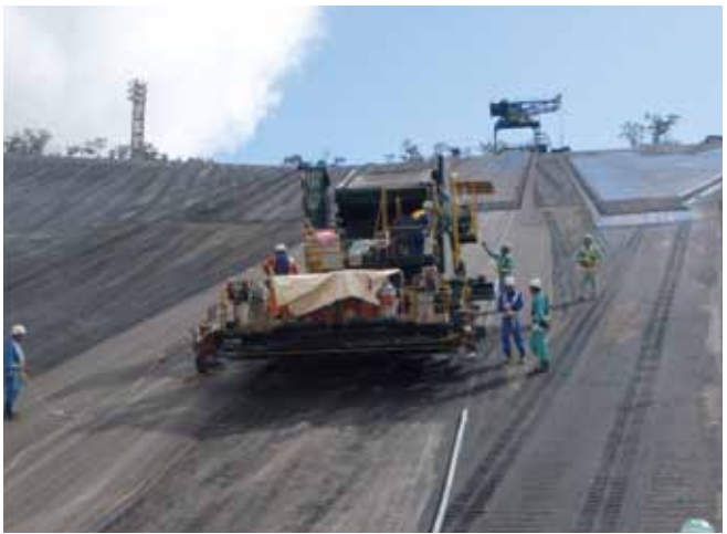
Laying test in progress (asphalt finisher with double tamper at work)
