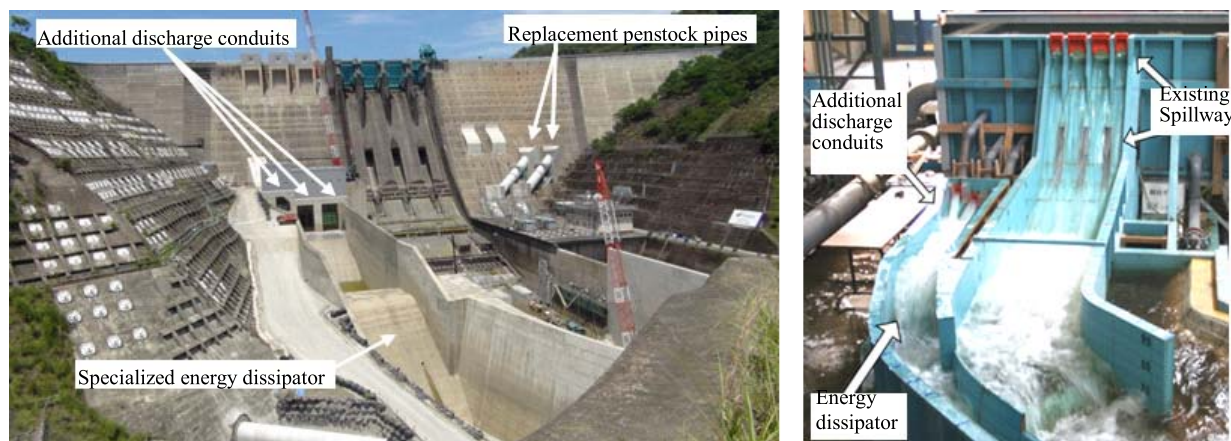
Figure 1: Construction situation of Tsuruda dam (June 2017) (left) and hydraulic model (right)
