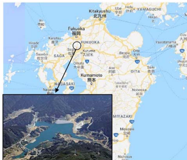
Figure 2: Location of Gokayama Dam
