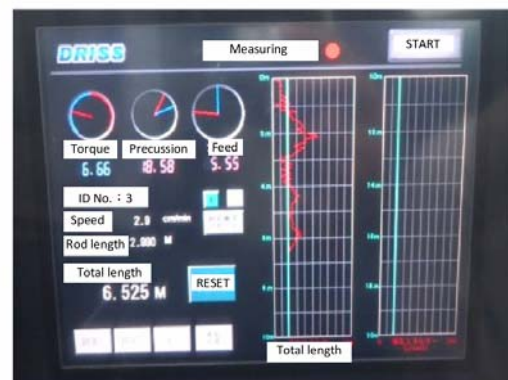
Figure 7: Drilling survey monitor in the operator room
