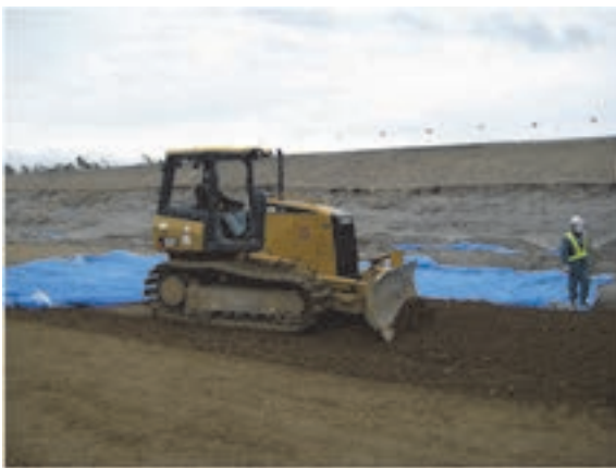
[3] Spreading of CSG
