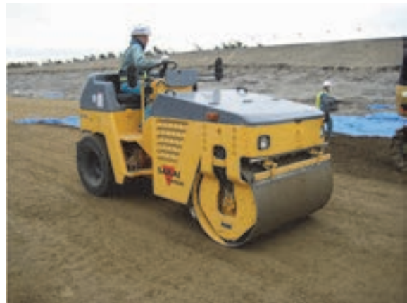
[4] Roller compaction
