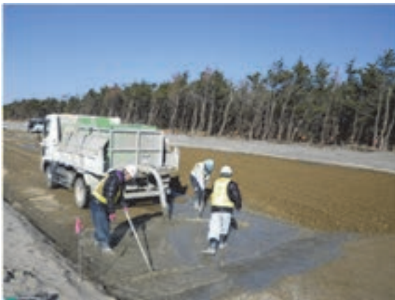
[1] Applying cement paste
