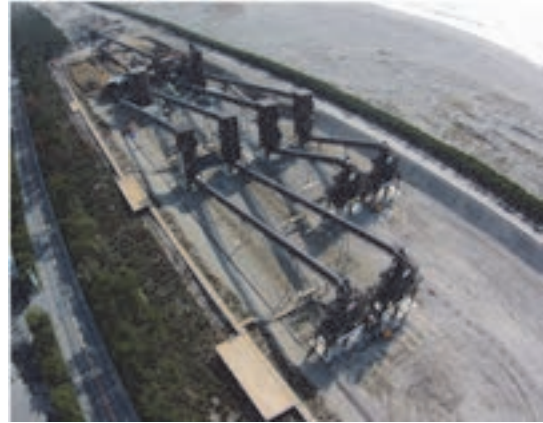
Figure 9. CSG mixing plant
