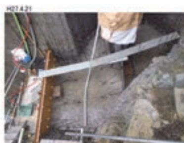
4th lift before concrete placing (EL195.5)
