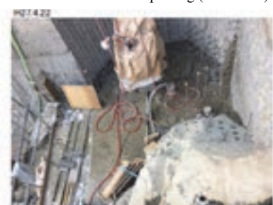
4th lift after concrete placing (EL196.25)
