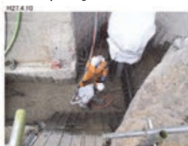
2nd lift before concrete placing (EL194.0)
