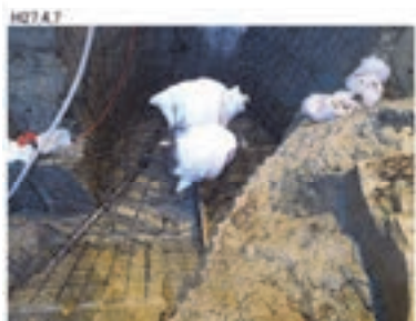
1st lift before concrete placing (EL193.3)
