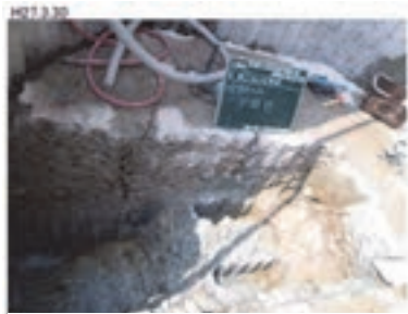
Deep cut in the rock foundation
