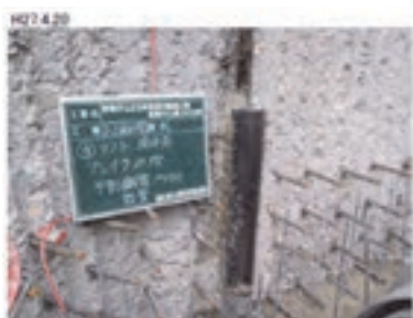
Joint bar setting to the old concrete body
