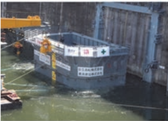
Figure 5. Towing to the dam body
