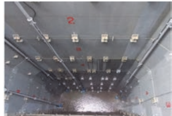
Figure 7. Inside the cofferdam after drainage
