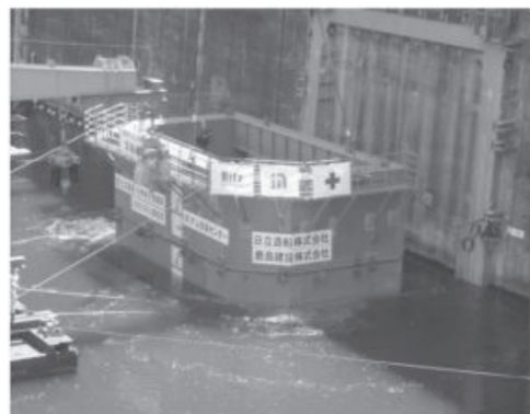
Picture 4 Floating type cofferdam installation
