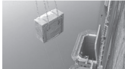
Picture 3 Transferring cut block
