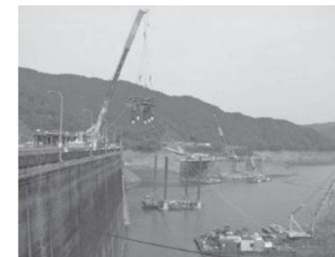
Picture 1 Installation of the large panel form
