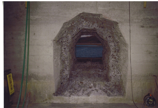
Figure-5 Dam body after drilling
