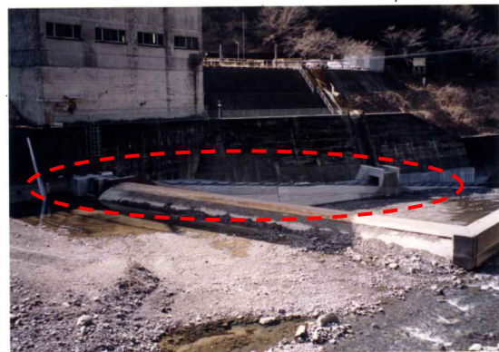
After construction of fishway
