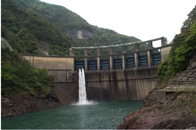
Figure-9 Discharging river maintenance flow from spillway gate of Futatsuno Dam
