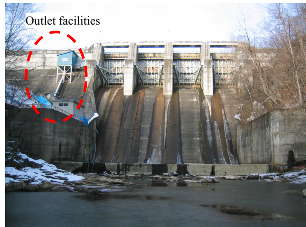
Figure-2 Kakkomi Dam and outlet facilities
