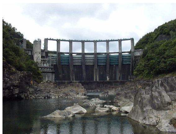
After discharging river maintenance flow Figure-8 River circumstances at Nanairo Dam
