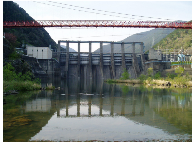
Figure-12 Downstream view of Akiha Dam and Akiha No.3 Power Plant
