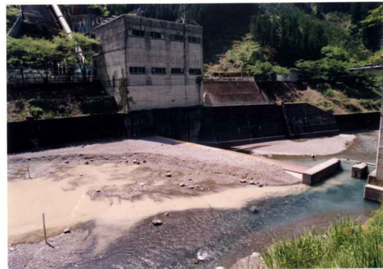
Before construction of fishway
