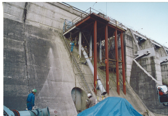
Figure-6 Installation works of outlet
