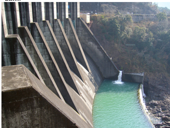
Figure-7 Discharging from outlet valve at Nanairo Dam
