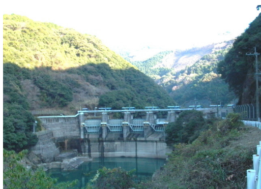
Photo 1 Emergency discharge equipment at Hitotsuse Dam
