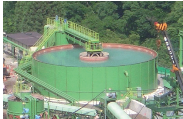
Photo 5. Installation of Turbid Water Treatment Plant
