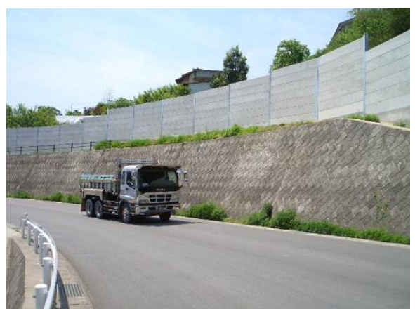
Photo 4. Installation of Noise Barriers (Top: before installation, Bottom: after installation)
