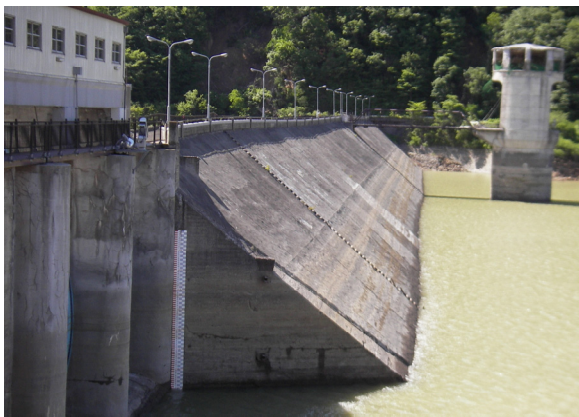
Photo.1 Concrete faced upstream slope on which no damage was found (Ishibuchi Dam) (Photographed by Public Works Research Institute (PWRI) on June 15, 2008)
