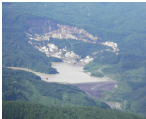
Photo.7 Huge landslides around the reservoir of Aratozawa Dam (Photographed by PWRI on June 15, 2008)
