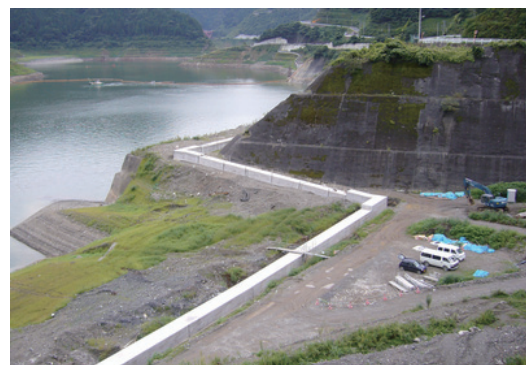
Fig.10 FRPM Pipe Section (2) (Completed with Concrete Cover)
