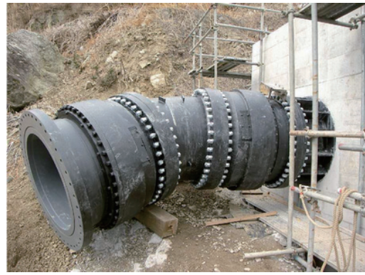
Fig.14 Suspended Pipe Section (4) (Rotation Joint)
