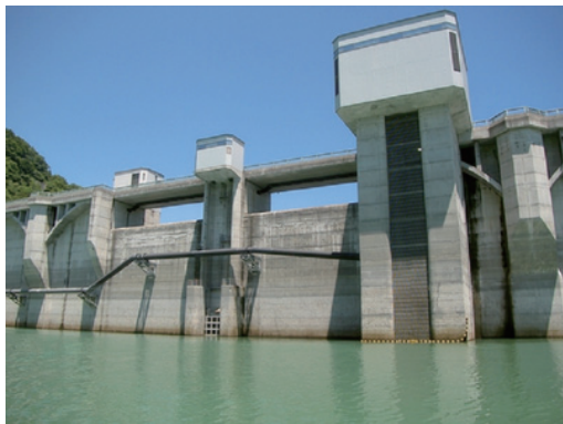
Fig.15 Outlet (1) (Intake Tower)
