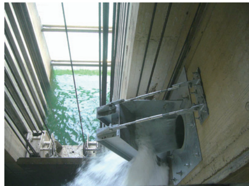
Fig.16 Outlet (2) (Inside the Intake Tower)
