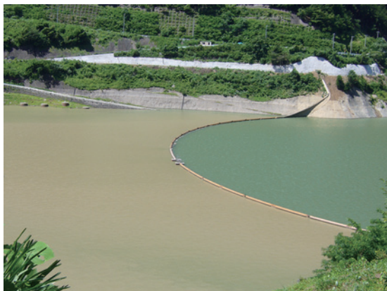
Fig.3 Floating Turbidity Curtain
