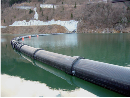
Fig.11 Suspended Pipe Section (1) (Before Submerging)
