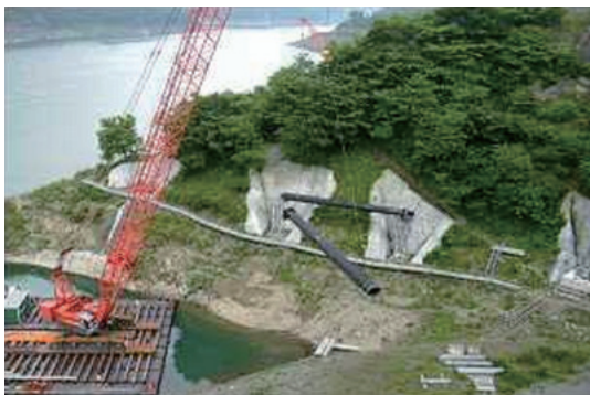
Fig.18 Construction Work (A Crane on the Pontoon)
