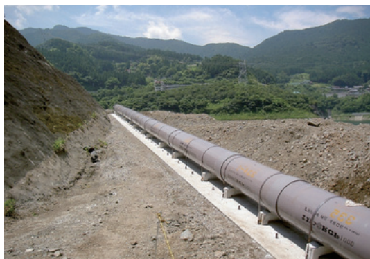
Fig.9 FRPM Pipe Section (1) (Under Construction)
