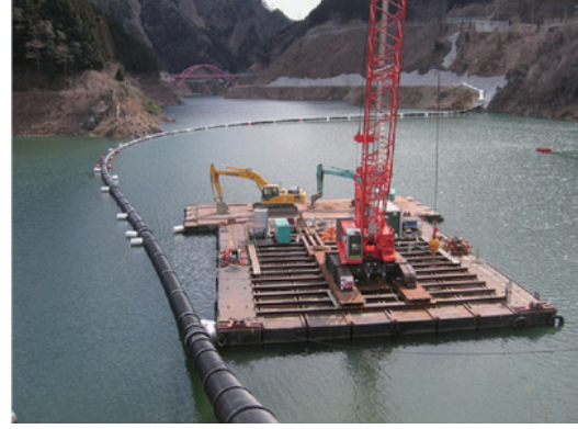
Fig.12 Suspended Pipe Section (2) (Construction Work)
