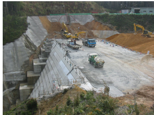
Photo 1.1 Execution of the Marsh Control Works at the Taiho Dam
