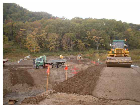
Photo 3.1. View of Execution of Cofferdam Upstream from the Tobetsu Dam
