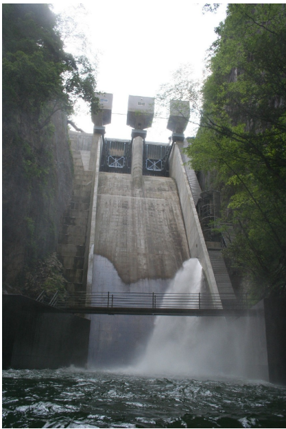
Fig.14 The Taishakugawa dam after rehabilitation
