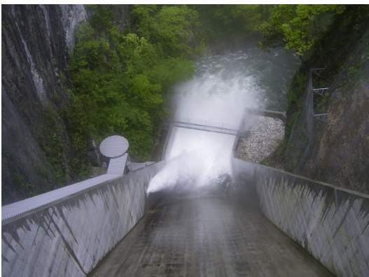
Fig. 10 Flush discharge at the dam site
