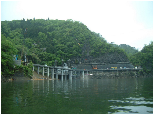
Fig. 6 Steel-made temporary road in the reservoir
