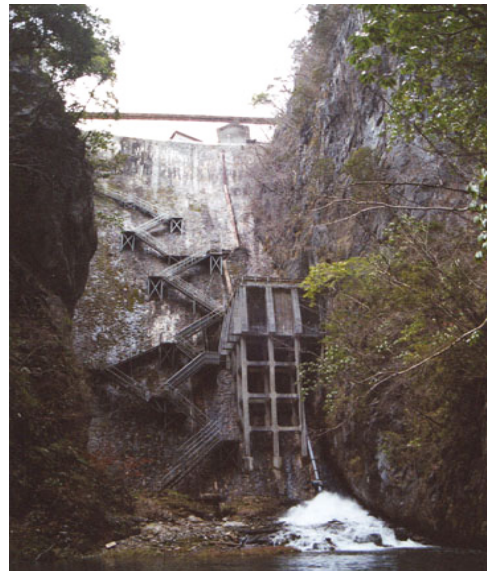
Fig. 1 The Taishakugawa dam (Before rehabilitation)
