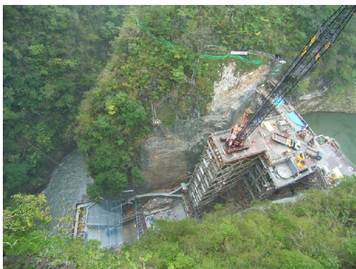
Fig. 7 Steel-made temporary stage on the downstream of the dam
