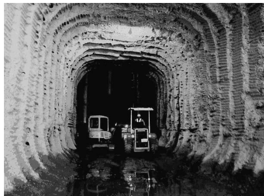
c) After tunneling
