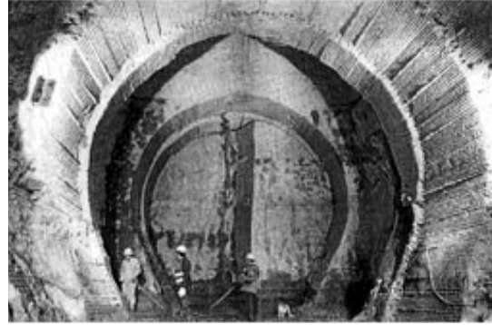
b) After tunneling
