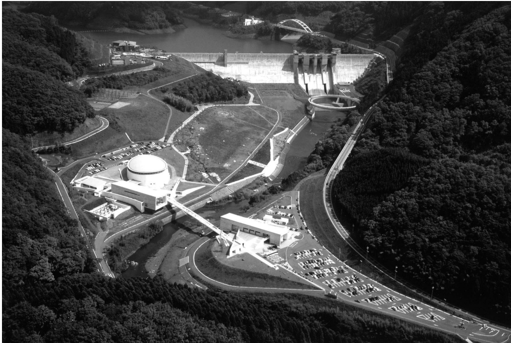
Photo 2 Hiyosh dam and springs park
