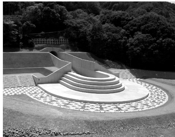
Photo-5 Current tunnel entrance
