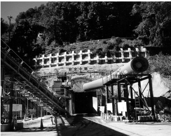
Photo-4 Construction of the tunnel entrance
