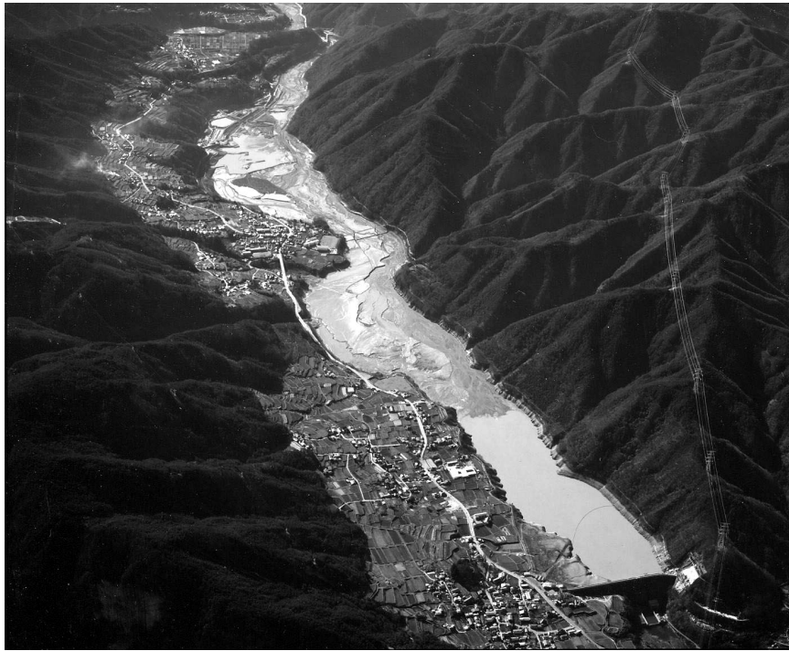
Photo-1 Miwa Dam during dewatering (the photo taken in 1989)
