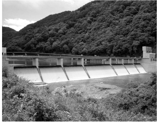
Photo-3 Current diversion weir
