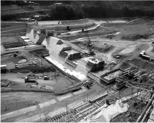
Photo-2 Construction of the diversion weir
