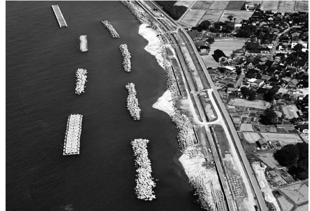
Photo 3 Establishment of offshore breakwaters (Yoshiwara District in Nyuzen Town)
