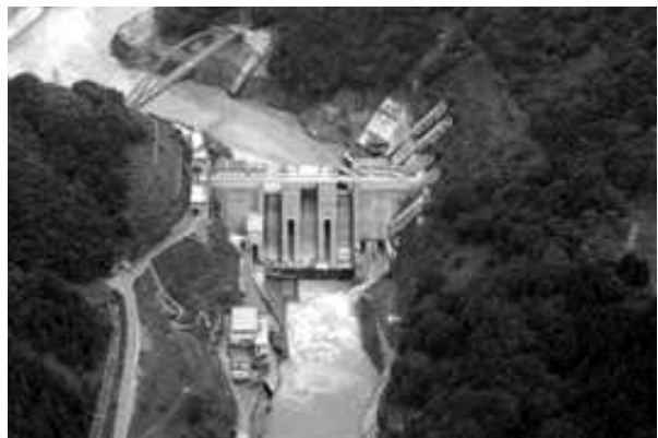
Photo 6 Unazuki Dam (during the drawdown operation)
