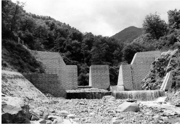
Photo 2 Establishment of slit-type sabo dam (Kokurobedani sabo-dam No.1)
