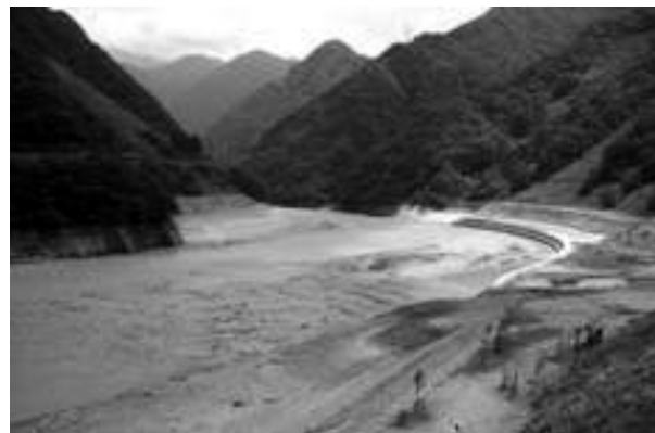
Photo 8 Unazuki Dam reservoir during the sediment flushing operation
