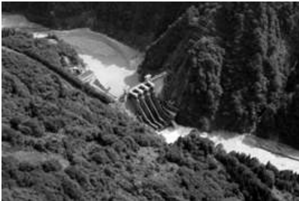
Photo 5 Dashidaira Dam (during the free flow operation)
