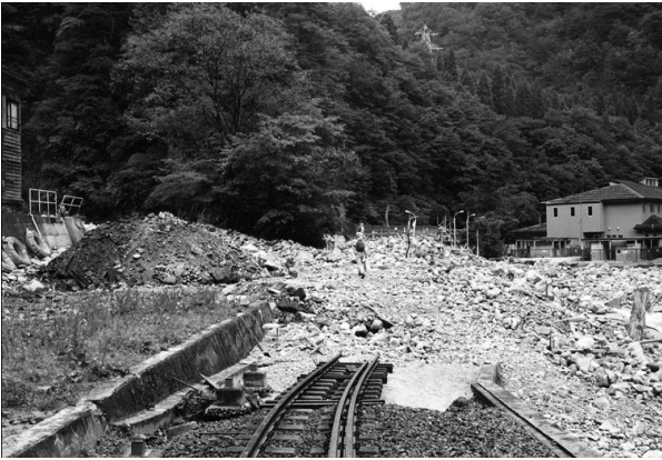
Photo 1 Damage inflicted on the Nekomata Station of the Kurobe Gorge Railway in July 1995
