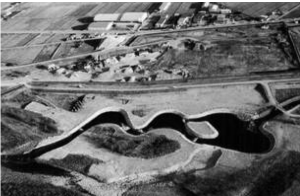
Photo 9 Evacuation facility for fish (resting water channel)
