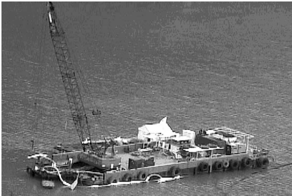
Photograph-1 Working barge with a crane to hang Hydro-J pipe
