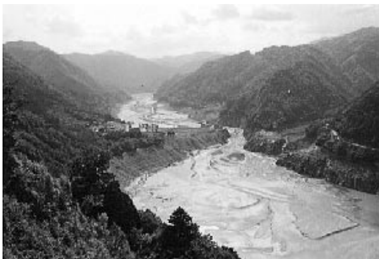
Photo 2 Condition of Deposited Sediment in the Makio Dam Reservoir (Upstream part of the reservoir bottom upgraded to the maximum of 15m by sediment deposit)
