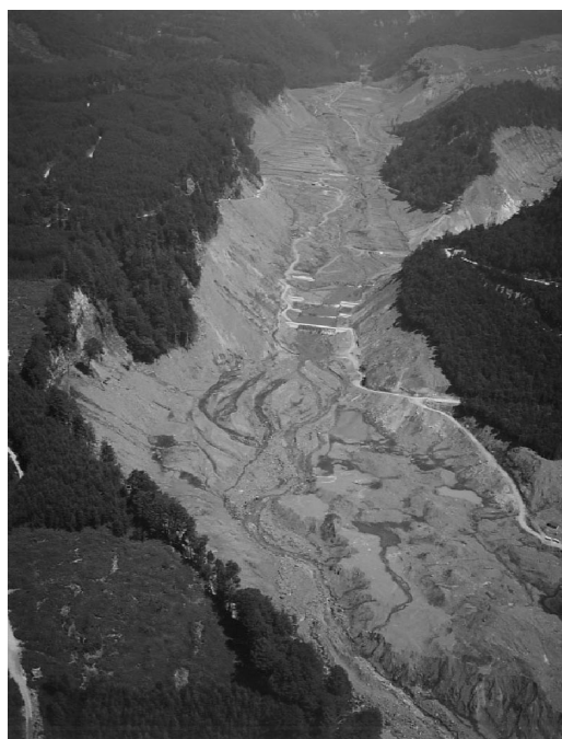
Photo 5 Condition of the Catchment Area immediately after the Earthquake
