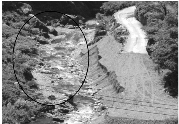
Photo 10 Present Riverbed Condition (May 2005) Note: Restoration of riverbed material can be seen.
