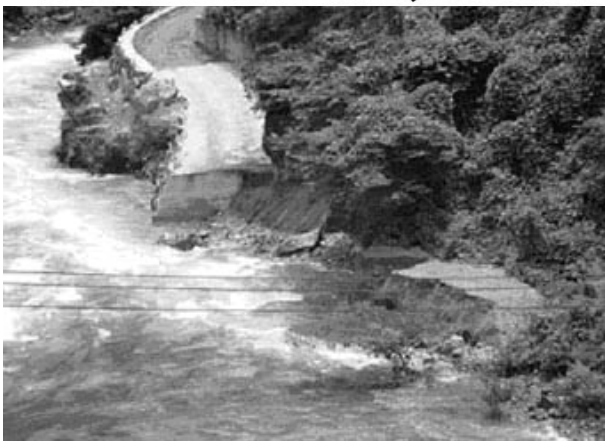
Photo 5 Sediment Transport by Reservoir Discharge
